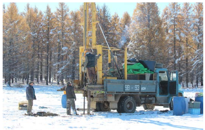
Figure 3. During the drilling work, Hangai mountain region, 2014.10.15
