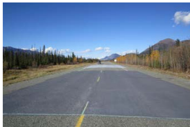
Figure 3. High albedo material test site, Alaska Highway, Yukon.
