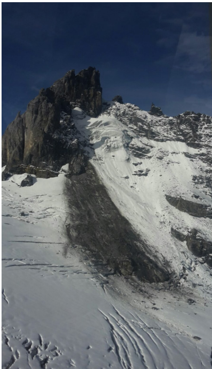
Figure 2. One of many rock fall events in the Swiss Alps during the summer 2015 heat wave: Spannort, September 2015 (Photograph Christian Schindler, Swiss Helicopter).
