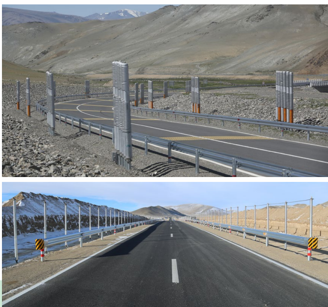
Fig. 36. Road embankments with looped thermosyphons in Buraat pass (top) and inclined thermosyphons in Tsagaannuur, both Western Mongolia.
