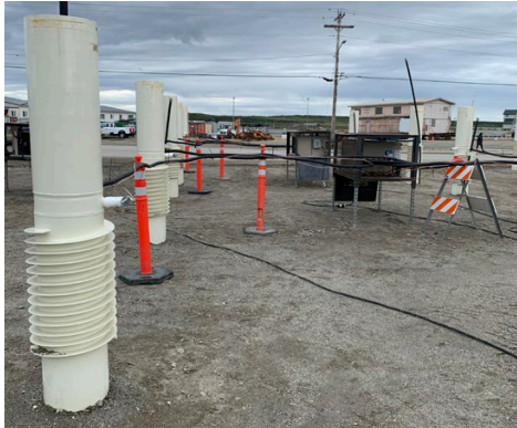
Hybrid Thermo Helix-Piles at the new general store, Kotzebue, AK.
