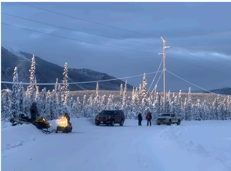
Using skidoos to compact snowbanks along the South McQuesten Road; an offshoot road of the Silver Trail used to access Eagle Gold Mine north of Mayo, YT.
