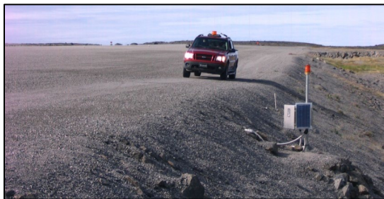
Figure 2. Engineering problem observed at Nunavik, Québec.
