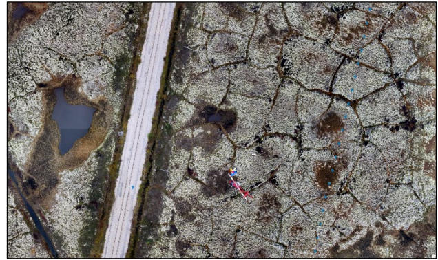
Figure 8. Drone image illustrating the extensive network of ice-wedge polygons that characterize the Barrens region and that intersect the railway embankment (Belcher site).
