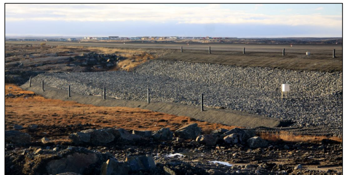
Figure 8. Application of ACE at Puvirnituk airstrip, Nunavik, Québec.
