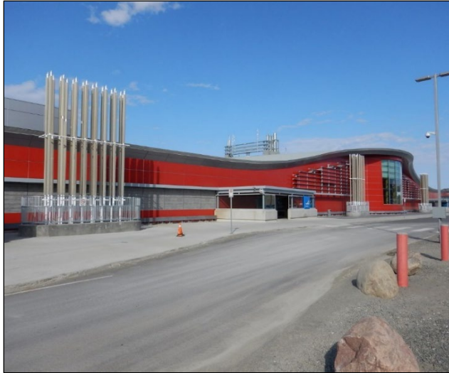
Figure 4. Front of the ATB showing three radiator banks.
