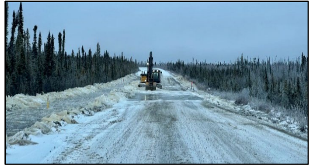
Figure 5. Surface icing adjacent and covering the Dempster Highway at km 20, November 2022. Photo by kind permission of L.P. Roy.
