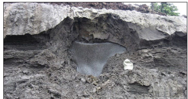
Figure 3. Ice wedge exposed in a road cut along the Dalton Highway, Alaska, USA. The baseball cap on the right provides the scale. All copyrights reserved to AKDOT.
