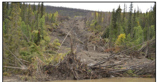
Figure 7. Landslides adjacent to Dempster Highway at km 244, July 2018. Photo by C.R. Burn.
