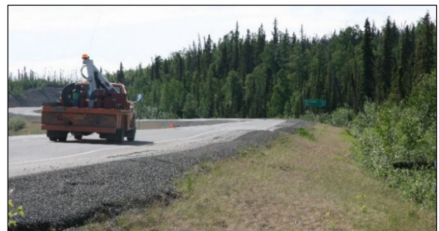
Figure 4. Localized thaw subsidence zones along the Dalton Highway, Alaska, USA, due to the degradation of ice wedges.
