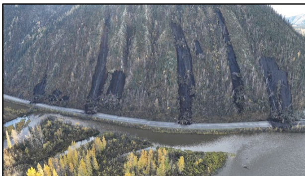
Figure 4. Photograph of September 22, 2022 active layer detachment slides impacting km 694 of the North Klondike Highway.
