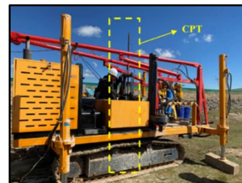
Figure 2. Cone penetration test equipment.
