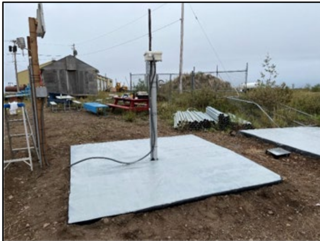
Figure 2. Evaluating freezing techniques - active liquid-filled thermosyphon in action.
