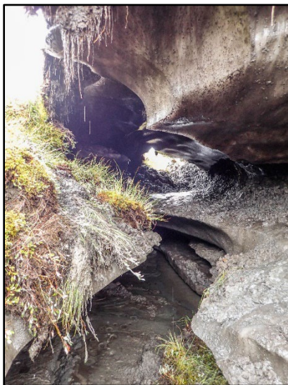
Figure 1. Thermo-erosional tunnel within ice wedge.
