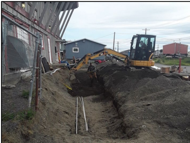
Figure 3. Quinhagak community members and ANTHC installing the flat-loop evaporator thermosyphon system.
